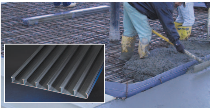
(above) SAFPLANK®, when turned upside down, serves as an excellent concrete forming system in applications where corrosion and weight are construction concerns.
