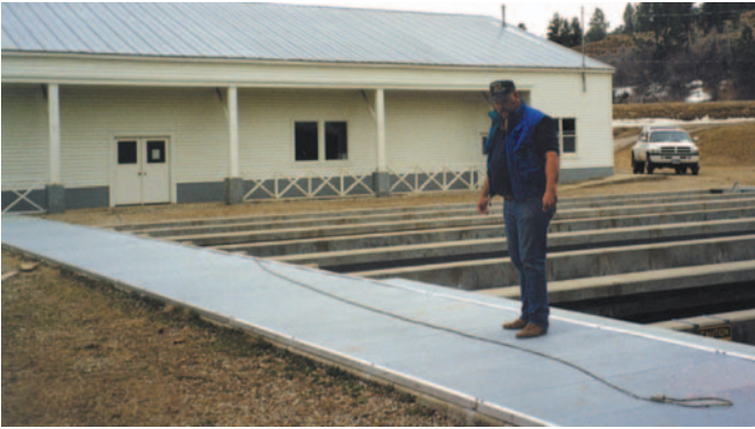
SAFPLANK® panels are used as tank covers at the Spring Creek Trout Hatchery in Lewistown, Montana. The lightweight panels allow easy access to the tanks and provide a safe walking surface for the staff.
