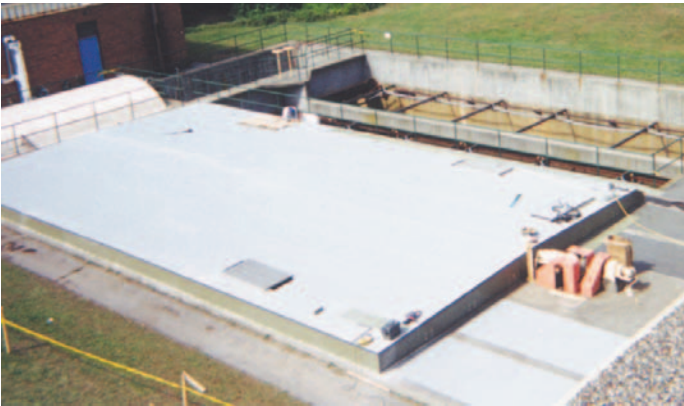
Odor control covers at a wastewater treatment plant in Smithfield, Rhode Island, will withstand the corrosive environment to provide years of trouble-free service.
